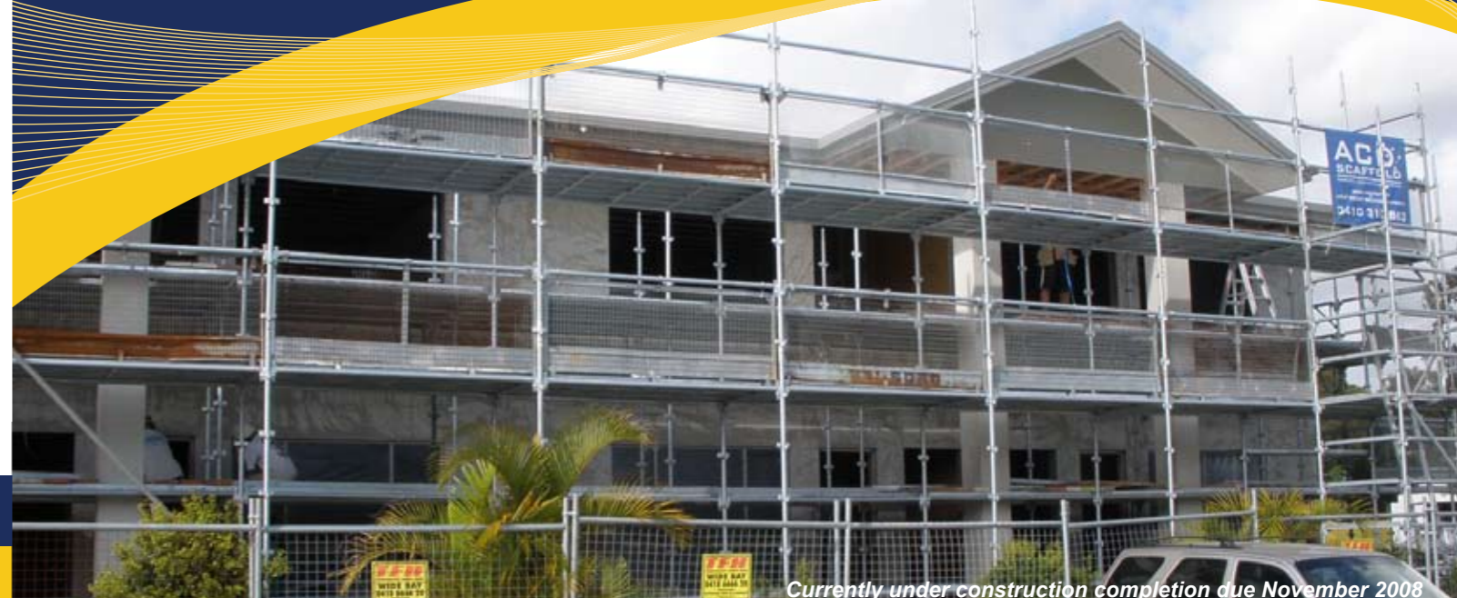
Currently under construction completion due November 2008
